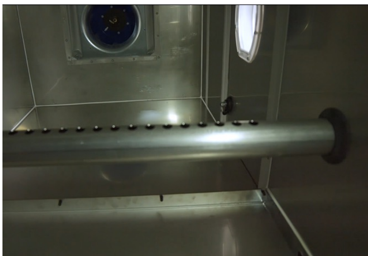
Figure 17. Steam Humidifier Section
