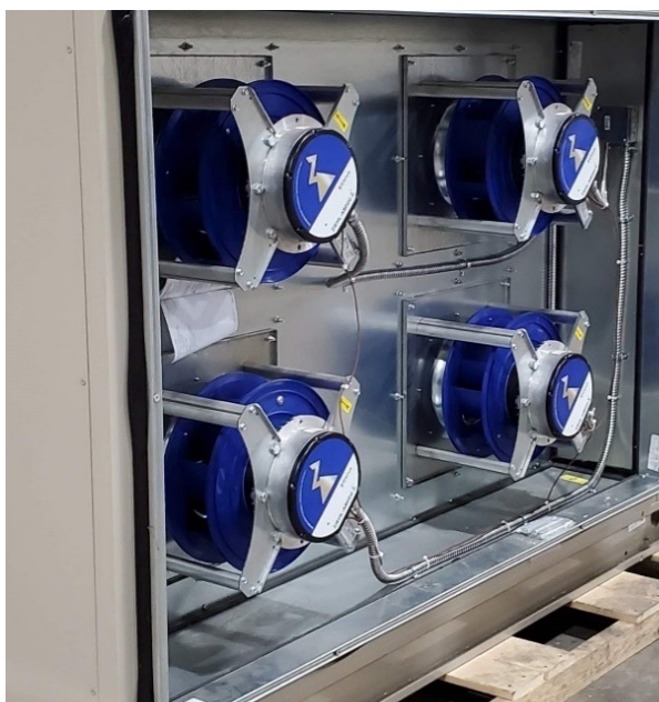
Figure 16a. EC Fans Section
