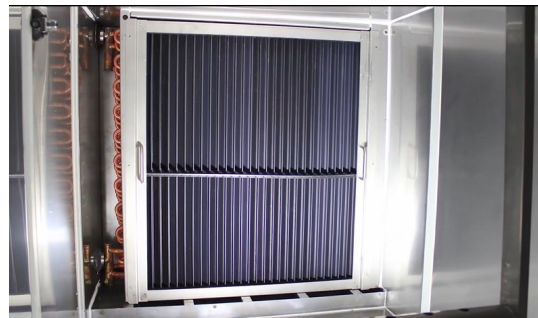
Figure 15. Coil Section with Droplet Eliminator as per DIN 1946-4
