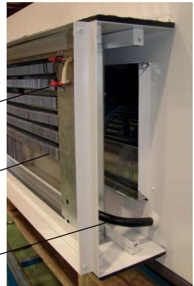
Then, unscrew the screw that fastens the electrical heaters' frame and take out by the rail, as shown in the following images.
